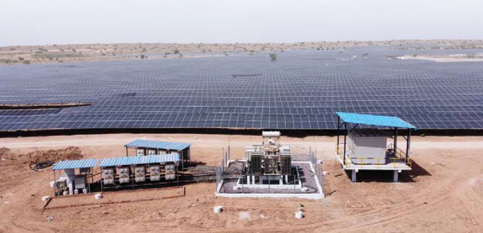
Assured Peak Power Project under SECI’s tranche-VII 300 MW Project with Solar-81 MW, Wind-322 MW and BESS-75MW, 150MWh
