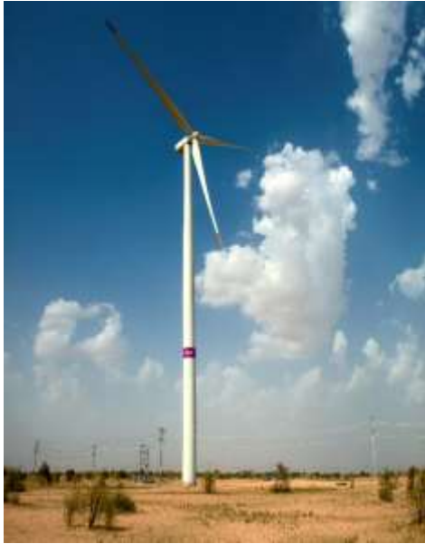
Wind Turbine in a 250 MW Project under SECI tender
