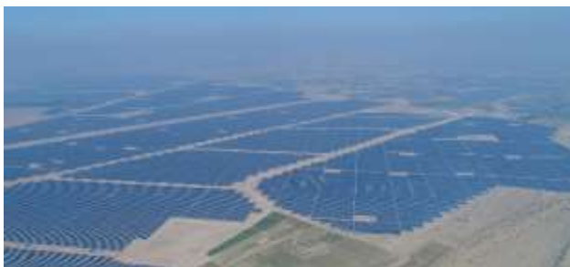
2245 MW Bhadla Solar Park, Rajasthan
