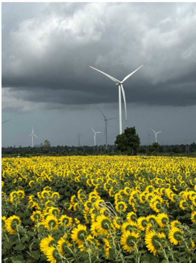
160 MW Blended Wind Power Project, Koppal, Karnataka
