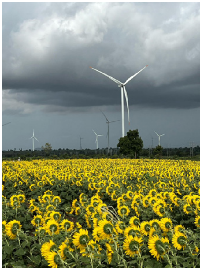
160 MW Blended Wind Power Project, Koppal, Karnataka
