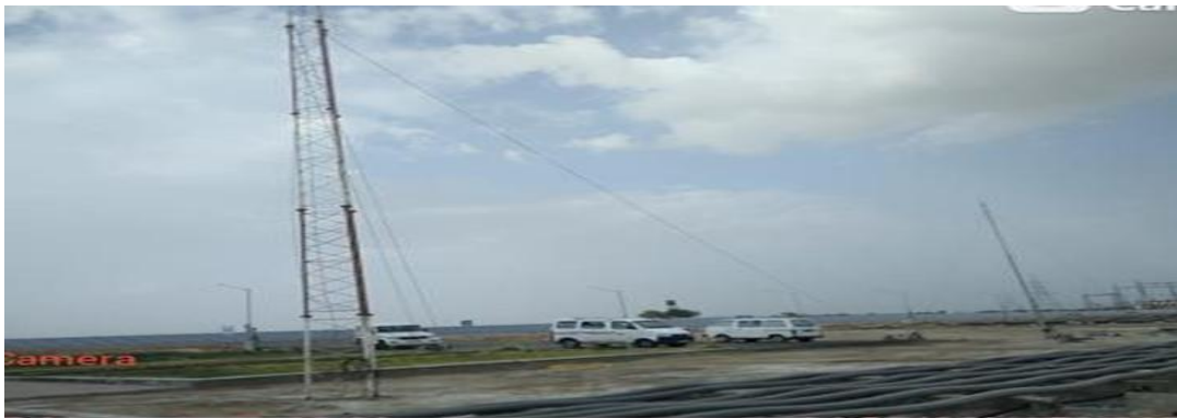
FIG: ROPE SUPPORT TO COMMUNICATION TOWER
