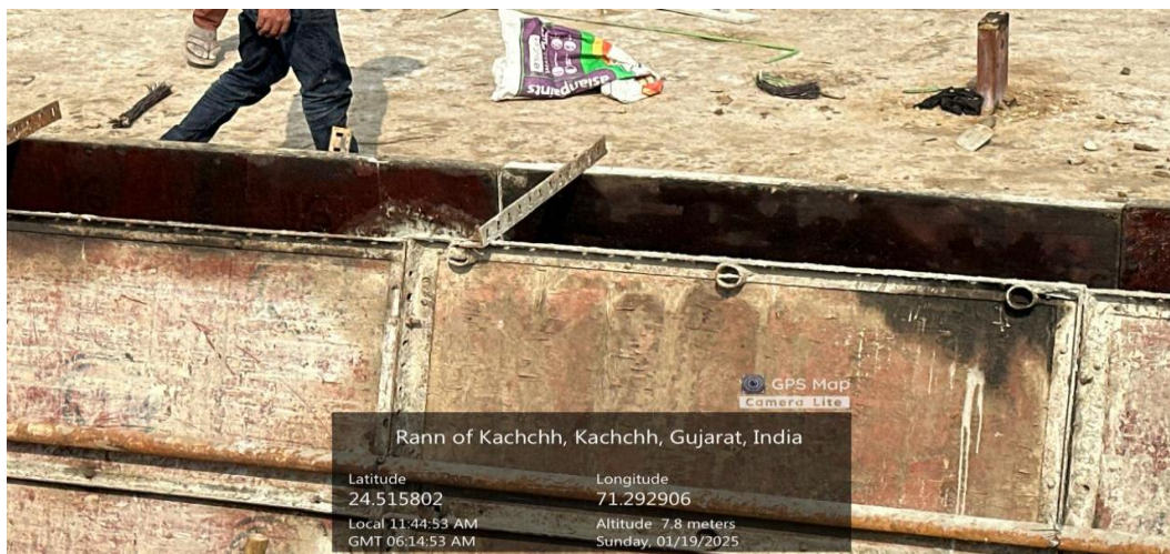
Photo 2.6 Retaining wall being constructed on upstream (plant side) toe of peripheral embankment
