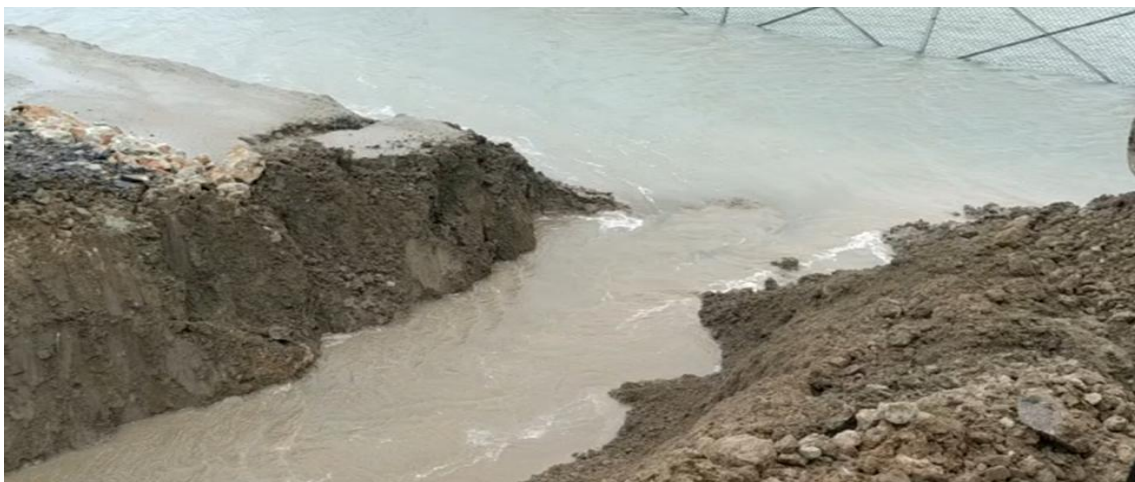
Photo 2.1 Cutting of Embankment to drain out the ponded water inside the solar park
